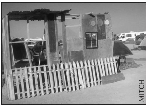
The Shack, under construction.
